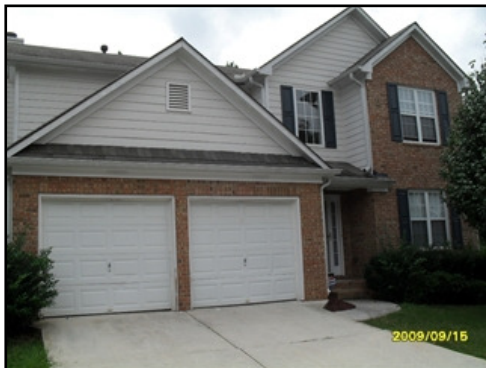
This is a house in Stone Mountain, Ga that we renovated in December 2009.
